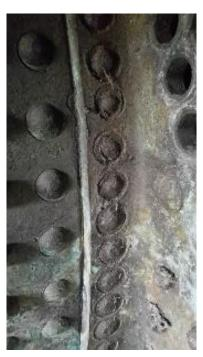
This sponsorship is for a set of three steel patch screws and includes the cost of removing the old rivet, tapping the hole, cutting a seat for the head of the patch screw, screwing in the patch screw and finally tooling over the head with a pneumatic tooling gun to effect a good seal.
